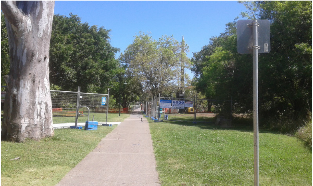
■ (a) Shared path before widening
