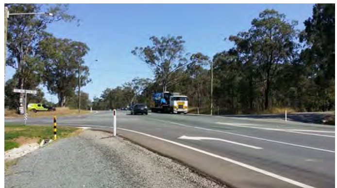
Photograph 13: St Aldwyn Road Intersection
