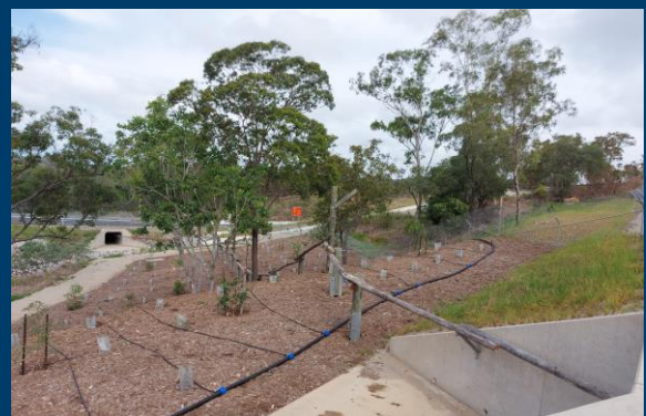
Pictured: Eton Range fauna underpass (Source: TMR)
