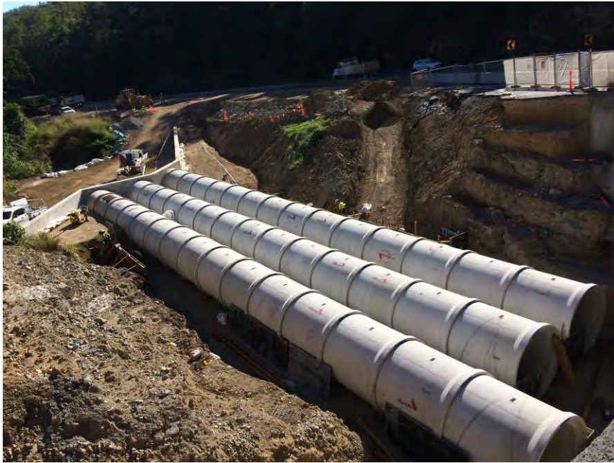
Figure 13: Culvert extension works at Cut Creek
