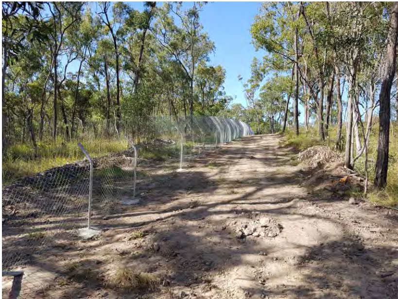
Figure 5: MC002 extension of fauna fence undertaken in February 2018
