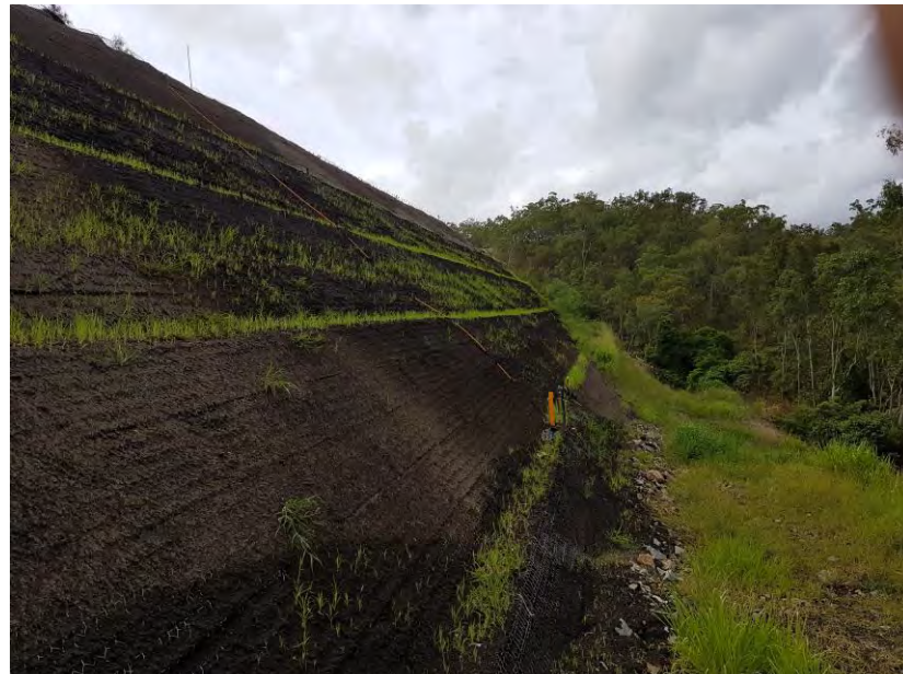
Figure 6: Permanent landscaping at reinforced earth embankment (REE 2)
