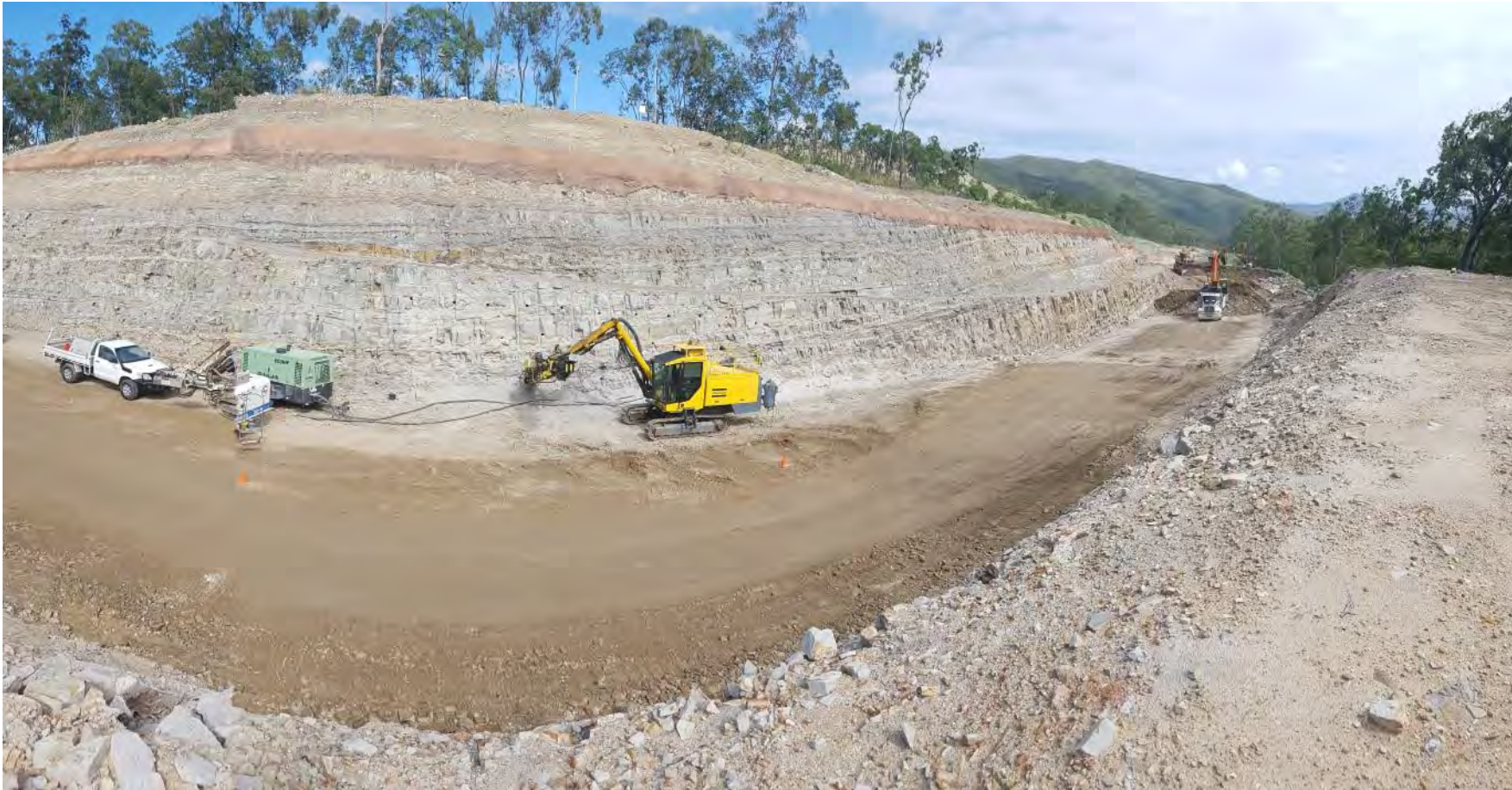
Figure 2: Significant earthworks, including rock hammering, at MCC002 cutting
