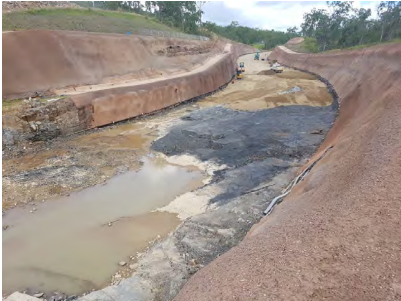
Figure 3: Shotcrete applied at the end of Cut 107
