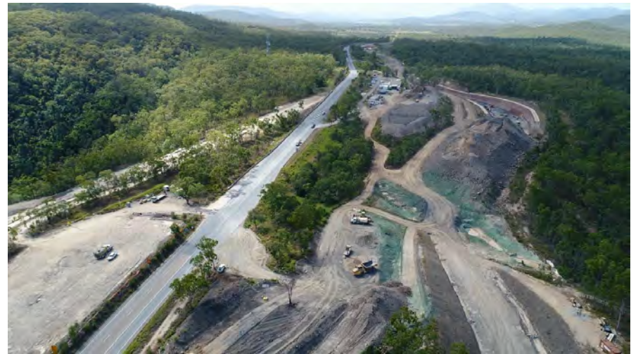
Figure 12: February 2018 drone footage of MC002 alignment, looking north
