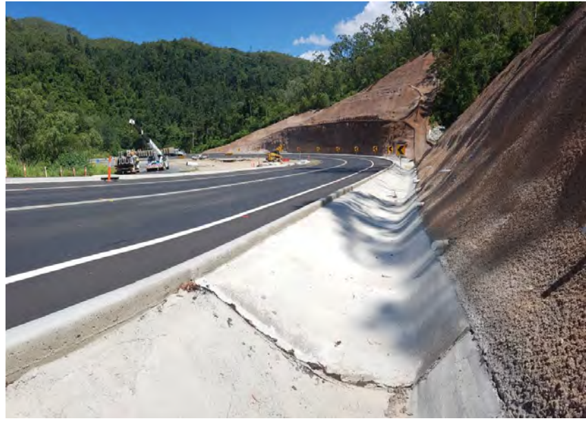
Figure 4: Permanent kerb and table drain works at Cut 215
