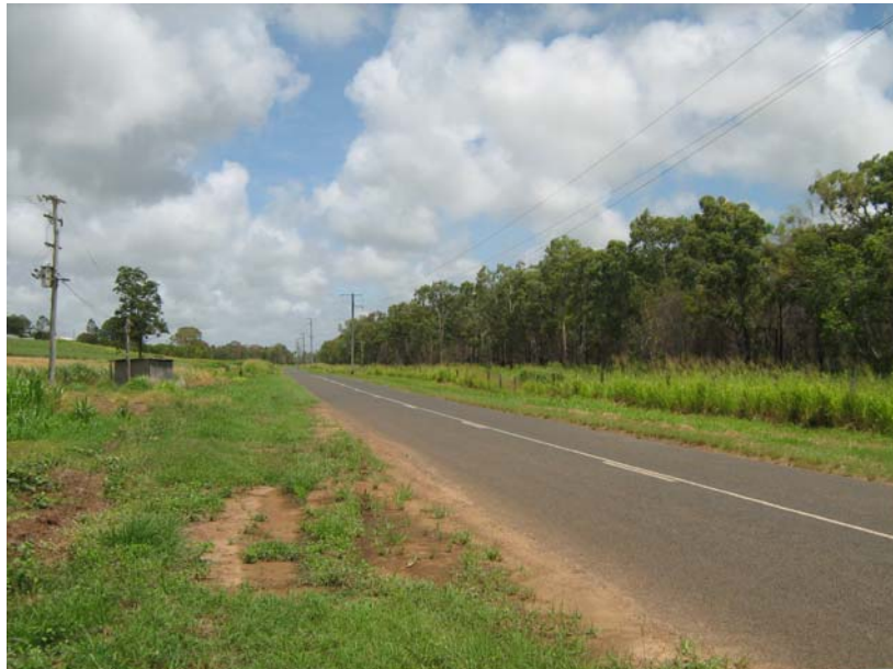
Figure 6 Gooburrum Road Closure
