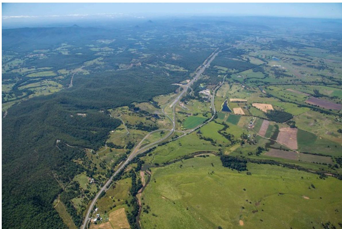
Figure 3 Completed Highway - Looking north to Woondum Interchange
