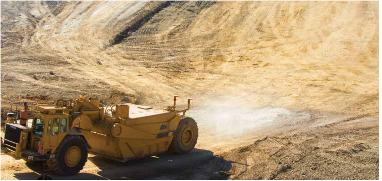
Dust suppression using large water trucks on open earthworks.
