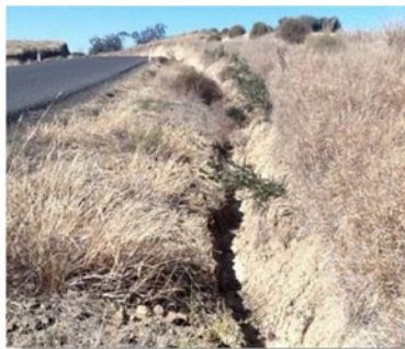
Eroded v-drain will continue to erode until vegetation establishes (unlikely in this instance) or invert reaches rock layer.
