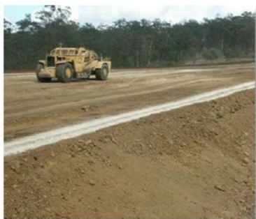
Ameliorant applied to outer embankment.
