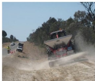
Ameliorant applied to cut batters.
