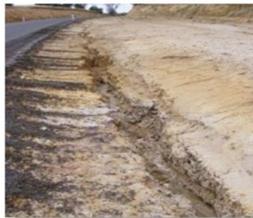
Eroded v-drain will continue to erode until vegetation establishes (unlikely in this instance) or invert reaches rock layer.
