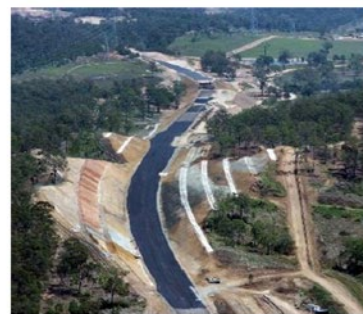
Ameliorant applied to embankment benches Source: Sinclair Knight Merz 2008.
