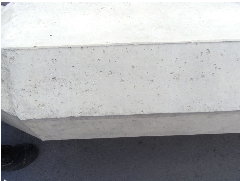
Figure 1: Acceptable Surface Finish following repair (Face C)
