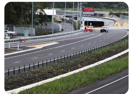
Figure 1: Wire rope roadside barrier
