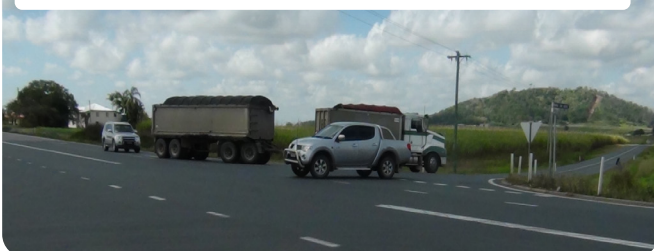
Auxiliary left-turn (AUL) lane on a major road
