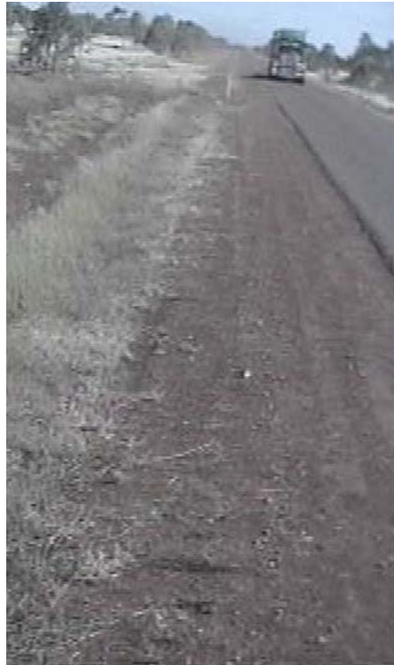
Figure 4.26 Example of road train operation on a single lane seal - Type 2 road trains remain wholly on the seal - approaching vehicles must therefore move off the seal
