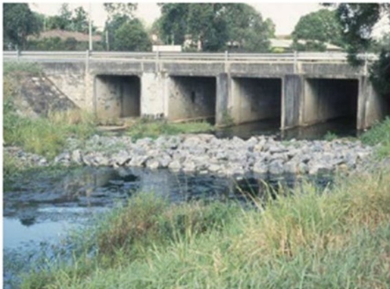
Figure 3.9 – Box Culverts with riprap
