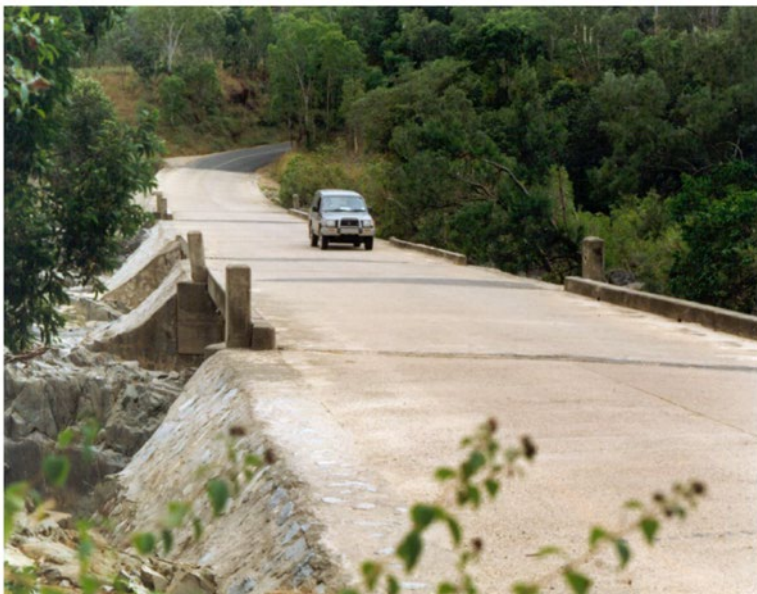
Figure 4.1 – Little Annan River floodway crossing
