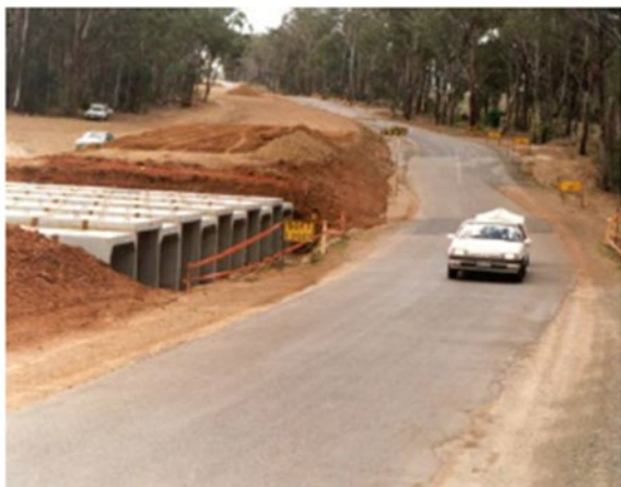
Figure 3.6.8 – Slab link box culvert under construction
