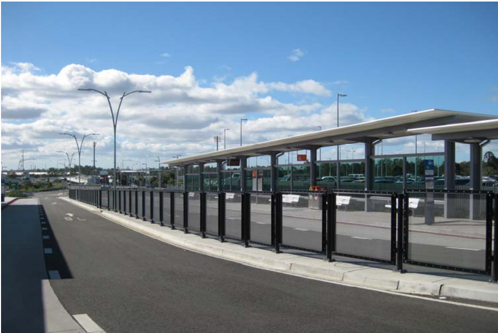
Figure C5-2: Improved surveillance through open style fencing
