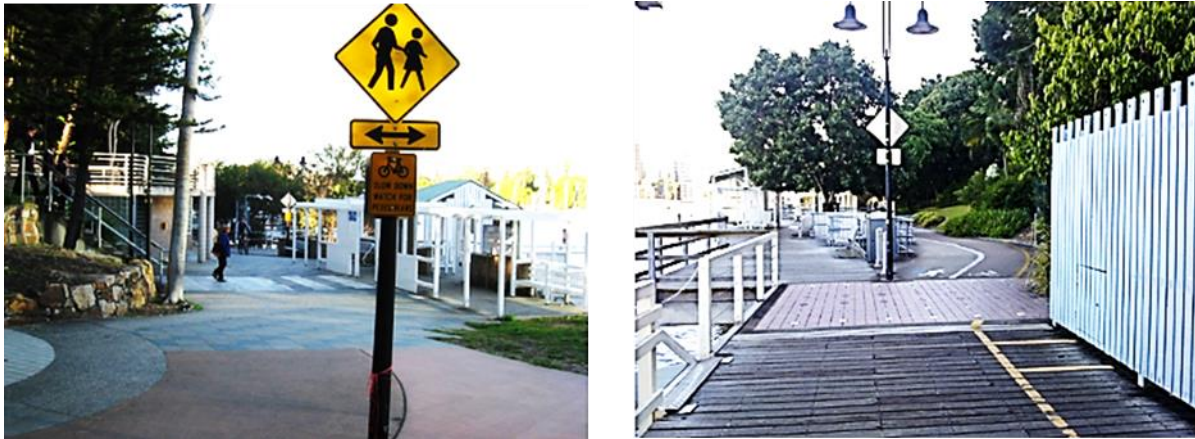
Figure 3.3 – Path safety issues due to broader design issues exacerbated by speed
