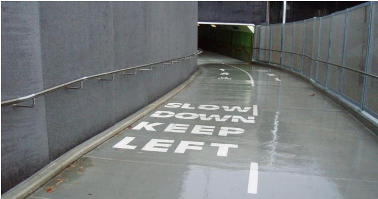
Figure 3.5(b) – Pavement markings use on a sight restricted corner to manage approach speed
