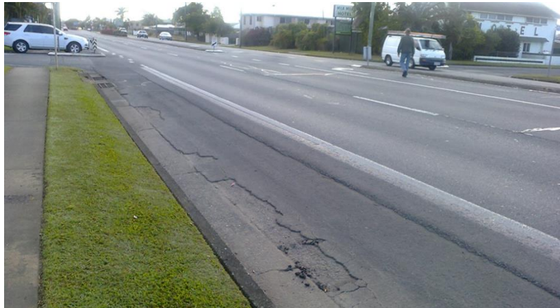
Figure 5(C) – Wearing course extent and proximity to traffic lanes
