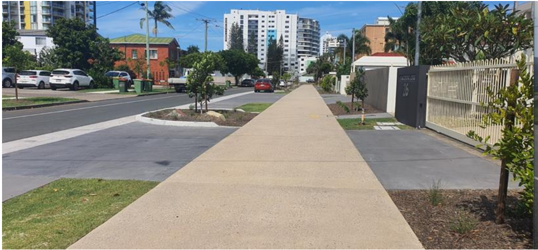
Figure 5(d) – Driveways to single residences that maintain good sight lines, promote low vehicle speeds and reinforce priority of path users.
