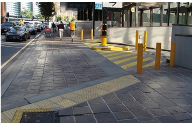
Figure 2.4(b) – Illustration of retrofitted treatments at driveway
